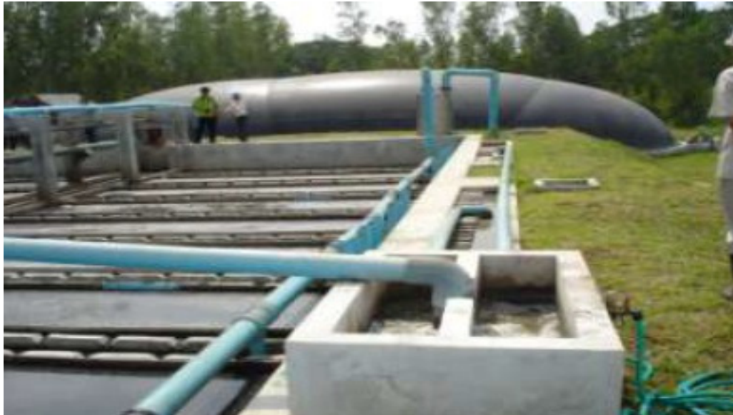
Figure 2.4 H-UASB (High suspension solid-Up-Flow Anaerobic Sludge Blanket)
